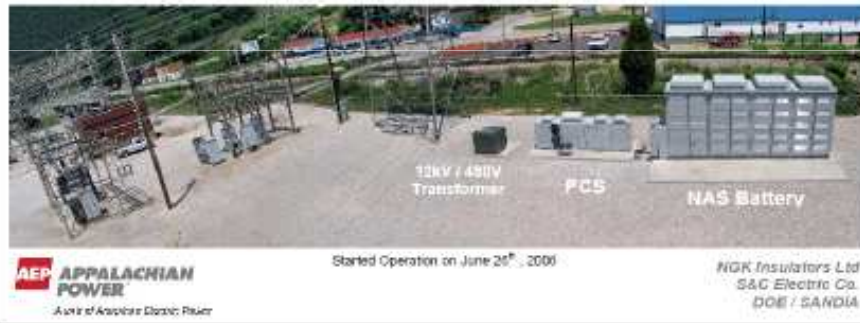
1.2 MW, 7.2 MWh Distributed Energy Storage System in Chemical Station, North Charleston
